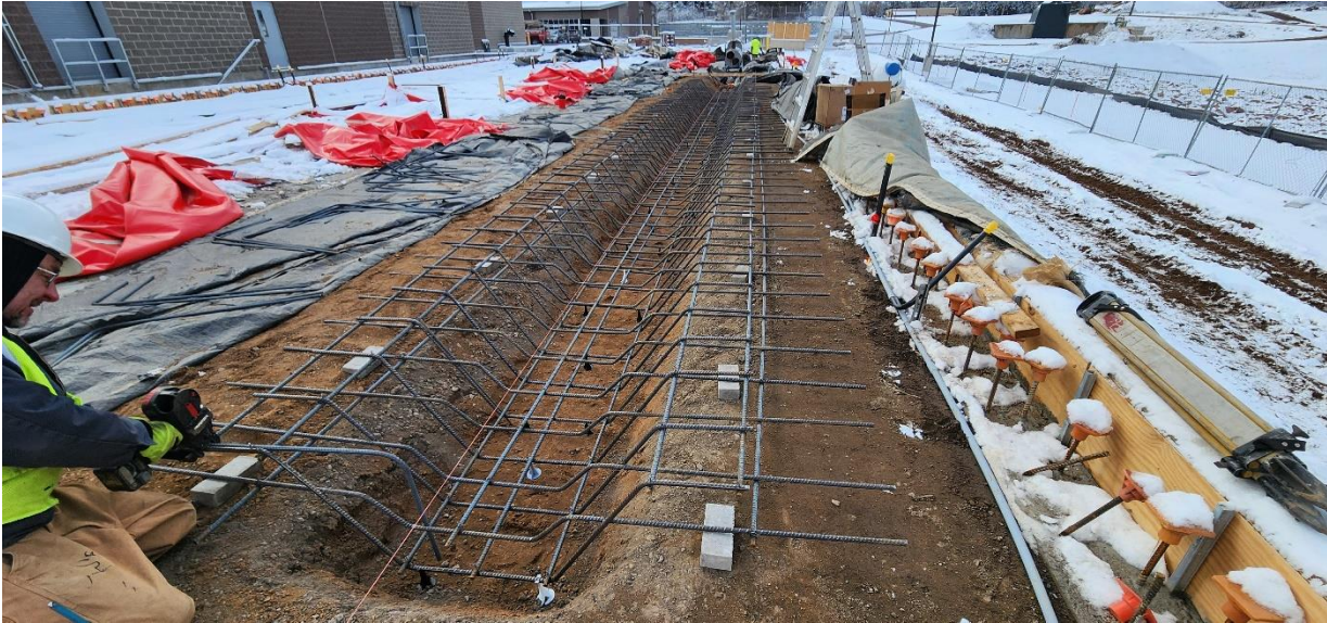
Rebar for north Structure 120 trench drain being installed.
