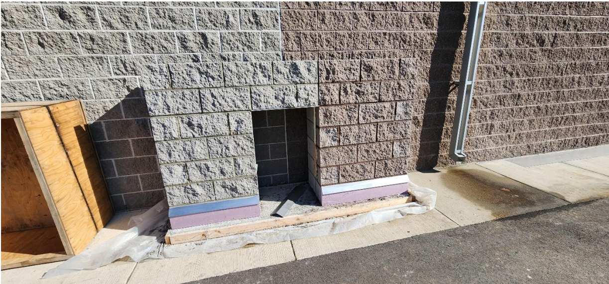
Masonry mock-up completed to show how new Structure 120 block compares to current Structure 100 block.
