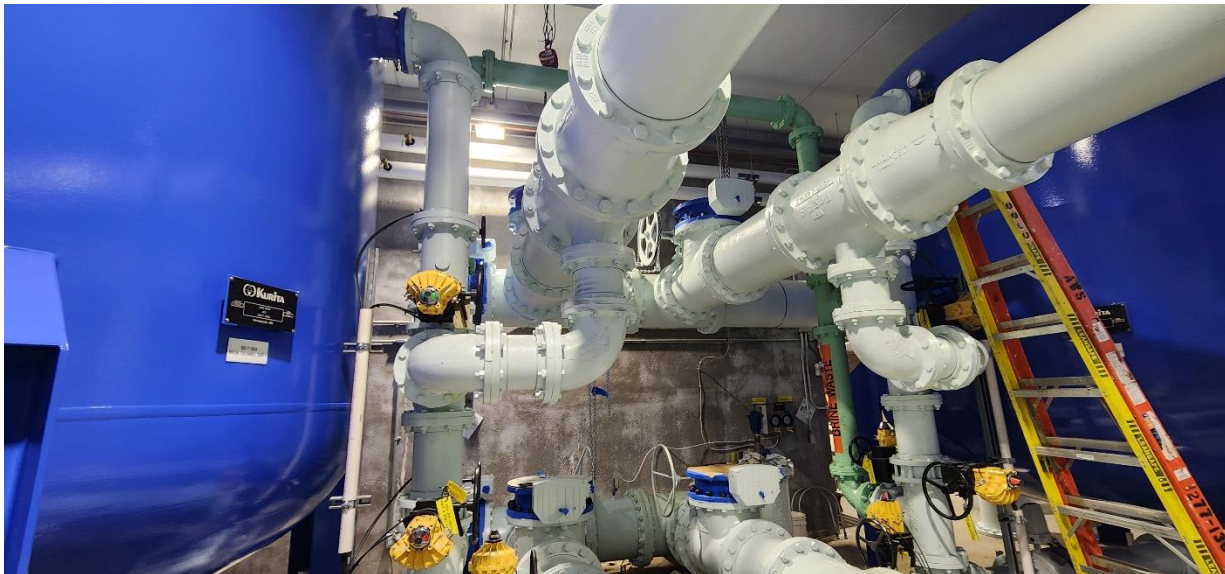
New 20" PFAs Effluent and Influent tie-ins installed with valves and painted.
