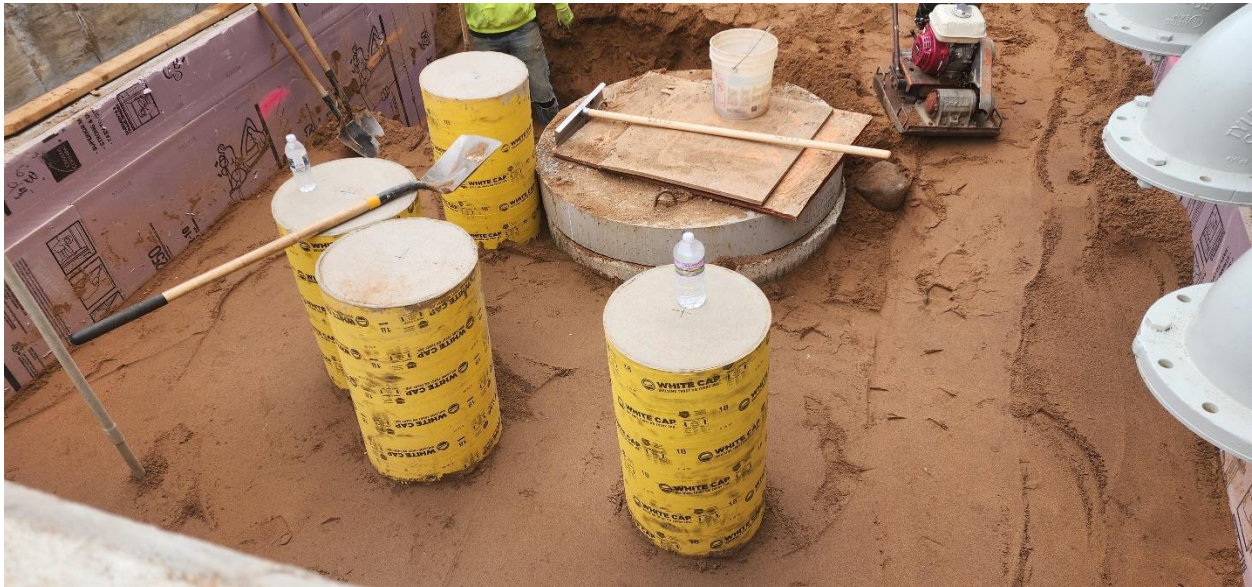
Lower pipe stand sonotubes poured between Structure 100 and Structure 120.
