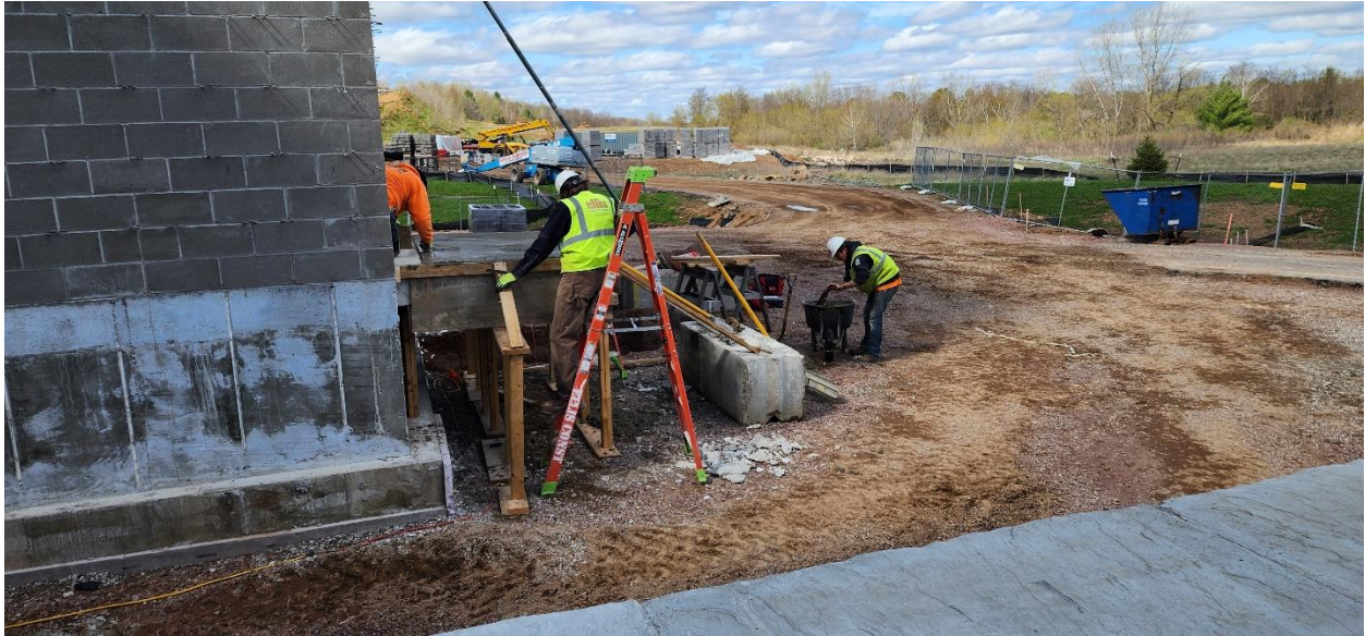
Ellis working on Structure 120 east cantilever stoop landing.
