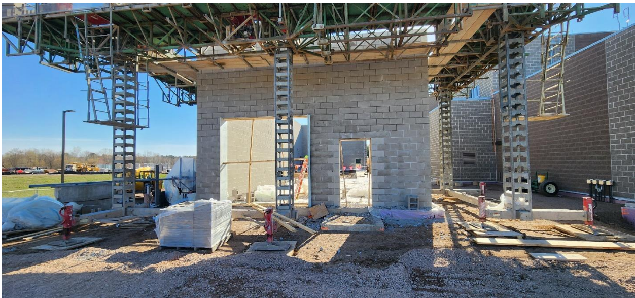
Masons working on west end of Structure 120 about halfway complete.
