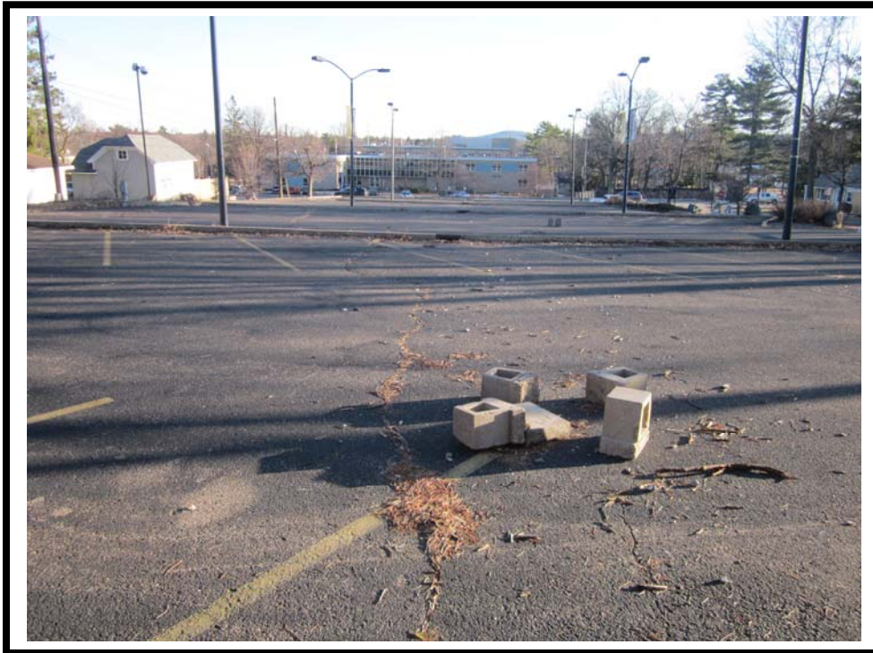
6. View of subject from the rear of the lot facing south.
