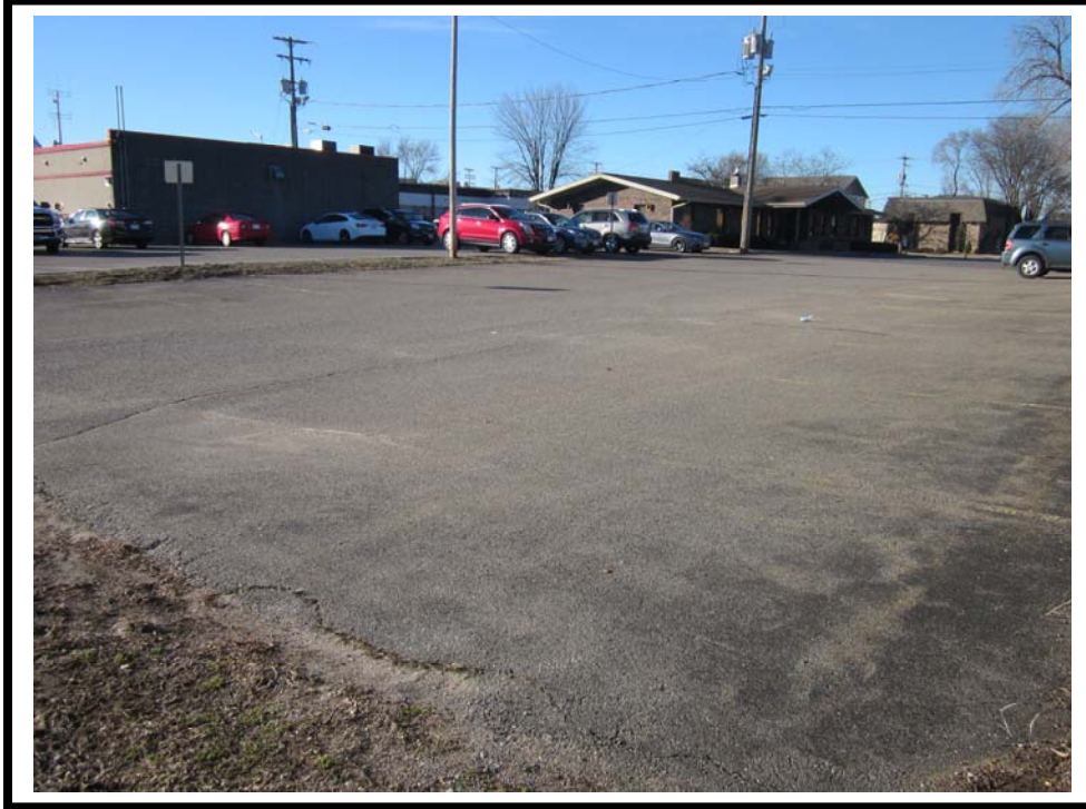
1. View of subject from the southeast corner facing northwest.
