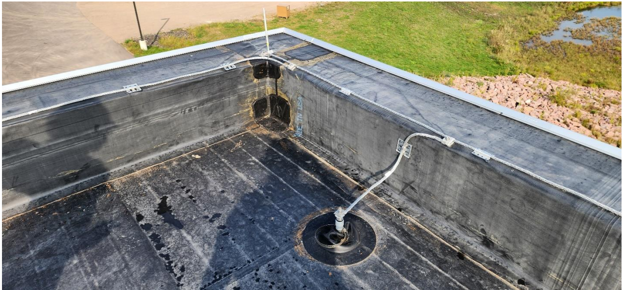
Structure 120 (PFAS Treatment Building) roof top lightning protection installed and connected.
