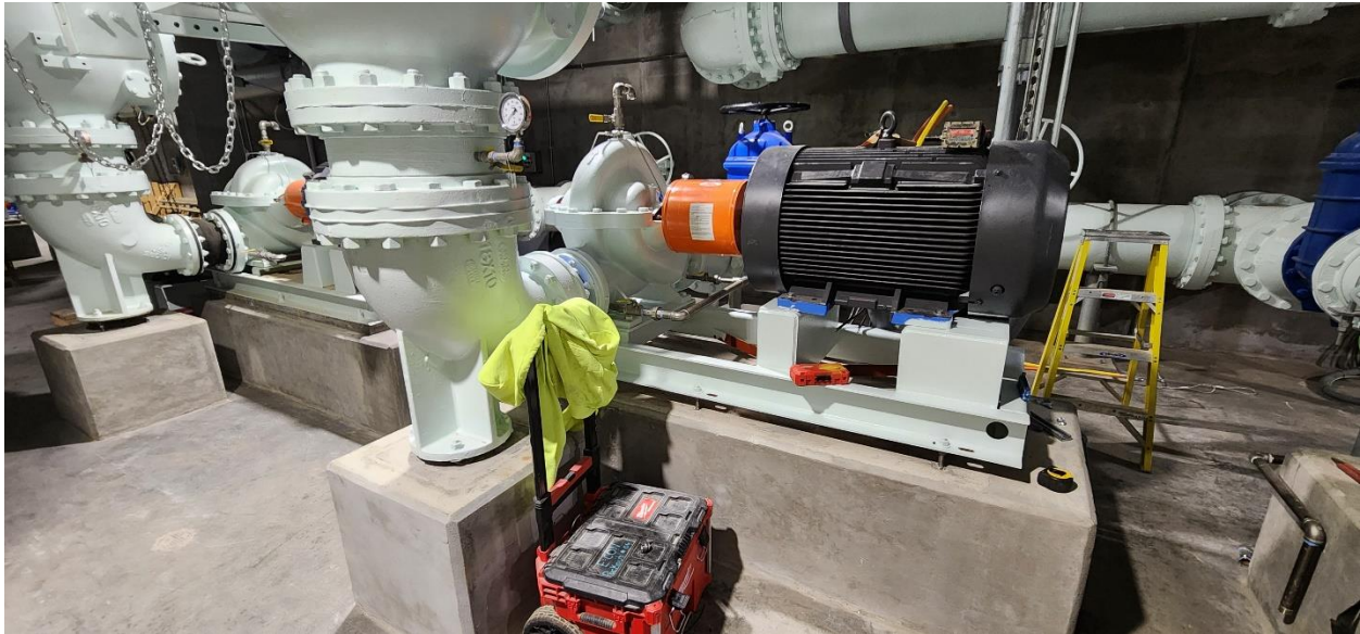
Structure 100 (Process Building) lower level Filtered Water Pump 2 installed.
