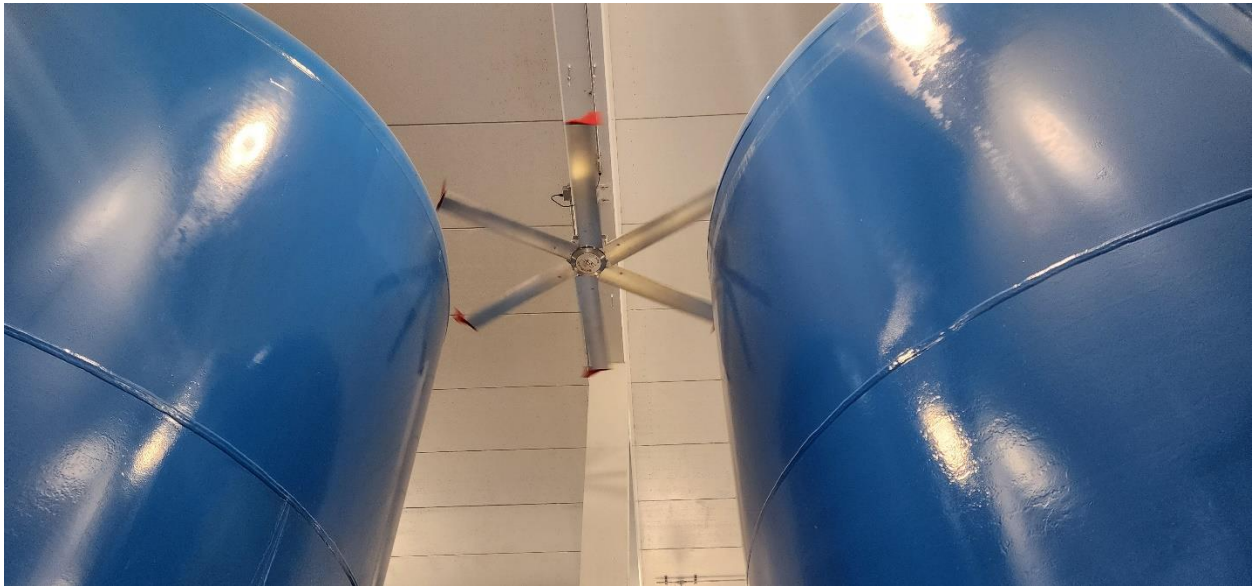
Structure 120 (PFAS Treatment Building) large ceiling fans & power/control installed.
