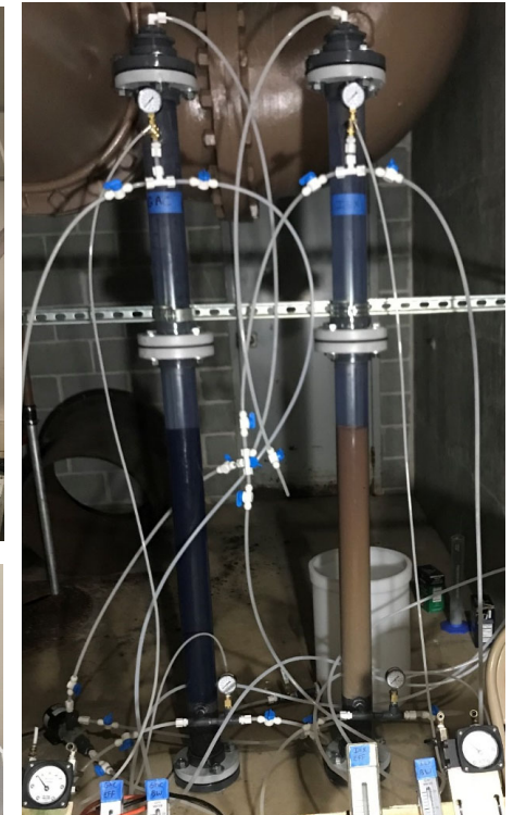
GAC (Left) & Ion Exchange (Right) Columns
