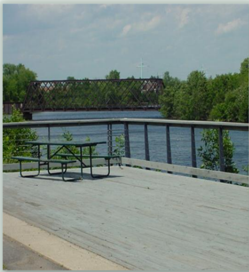
RAIL ROAD BRIDGE
