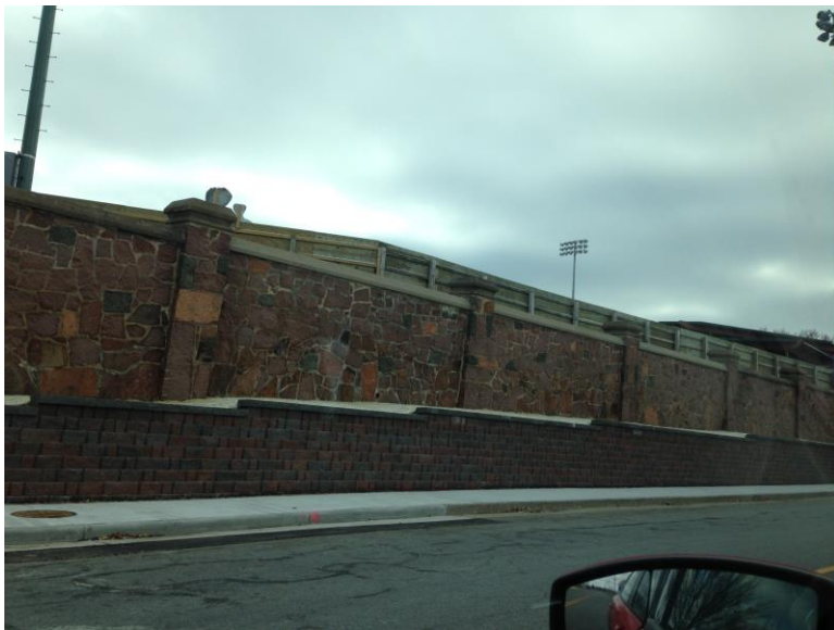
After – with sidewalk and rebuilt retaining wall
