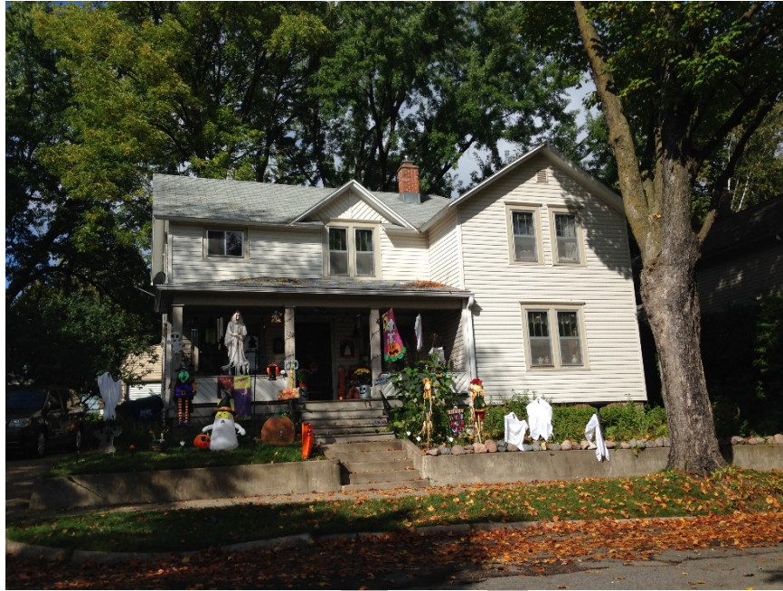
120 N. 7 th Avenue – Before
