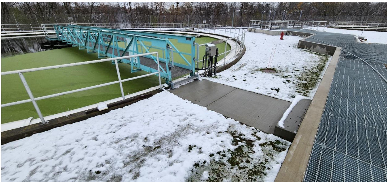
Step placed to access catwalk on Structure 530 (Secondary Clarifier 3).
