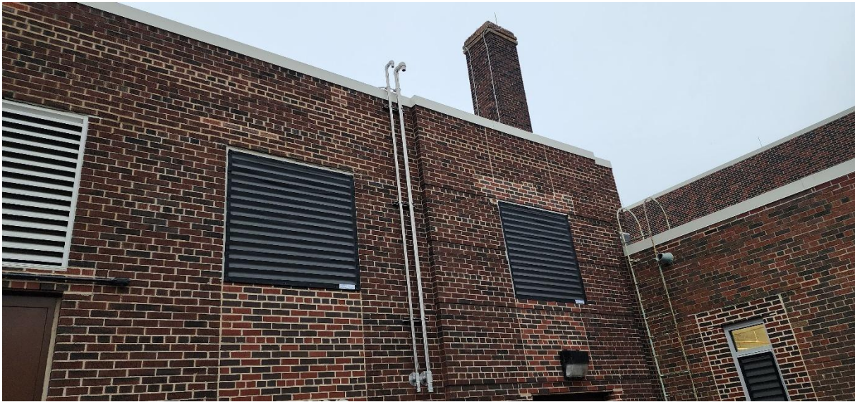
Screens placed on louvres around Structure 100 (Main Building).
