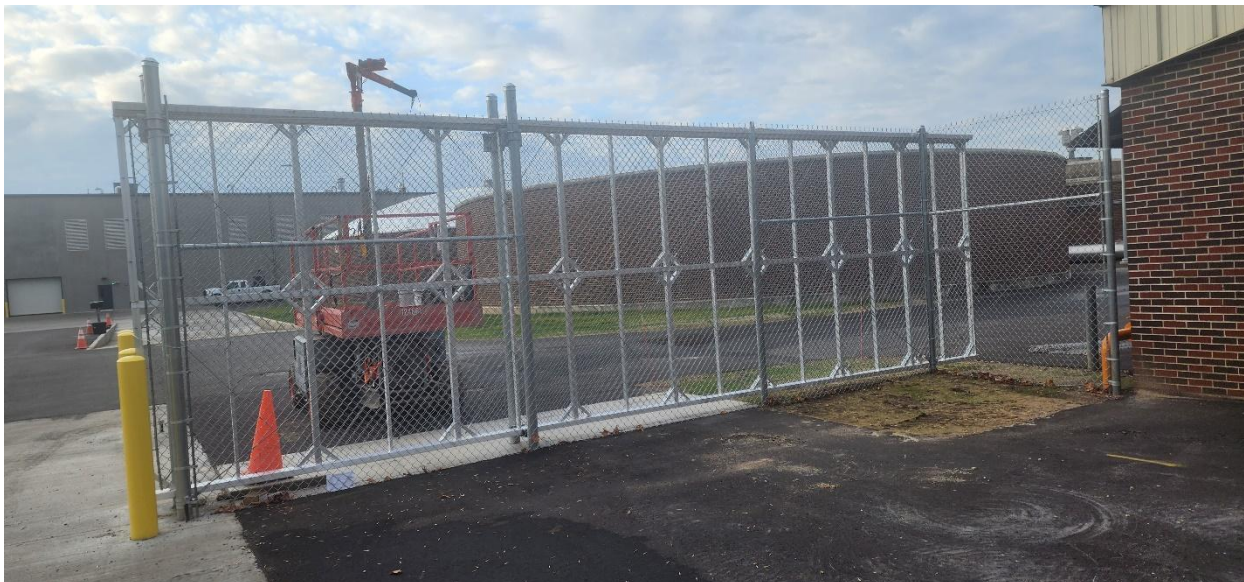
New east gate near Structure 110 (Vehicle Storage Garage).
