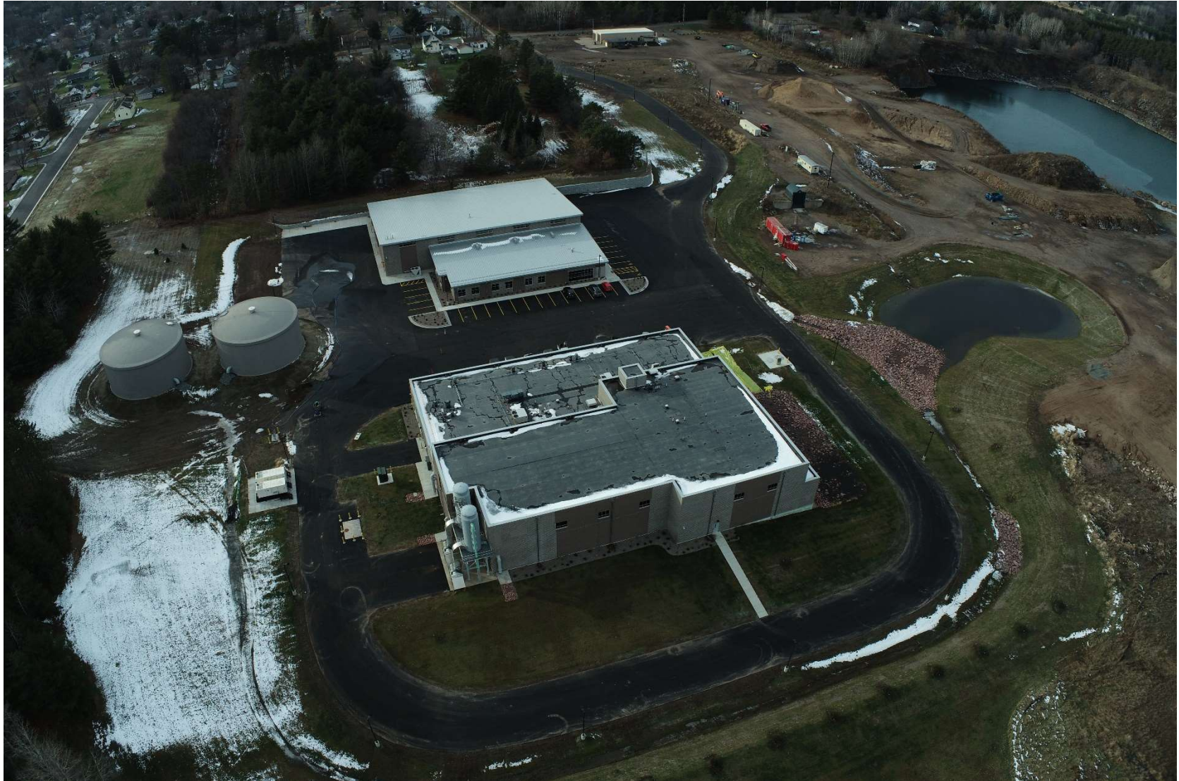
Aerial of Site Taken November 28, 2022
