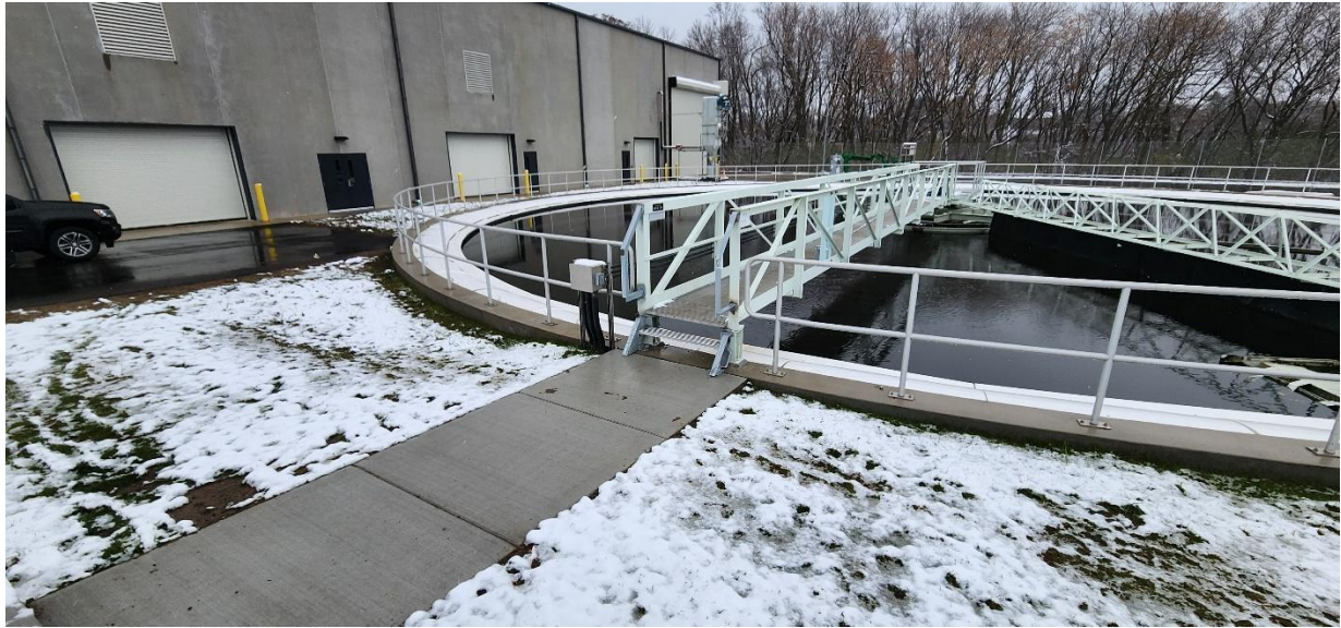
Step also placed to access catwalk on Structure 540 (Secondary Clarifier 4)
