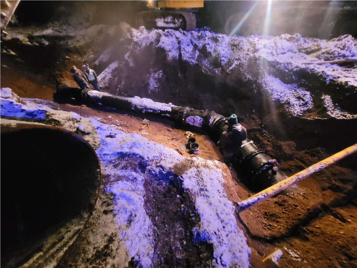
Final Treated Water Main Connection to the Cities Water Distribution System
