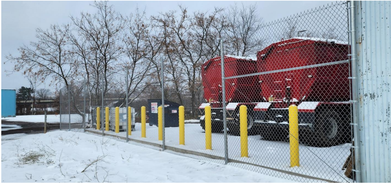
Fencing complete around Structure 120 (Administration Building).
