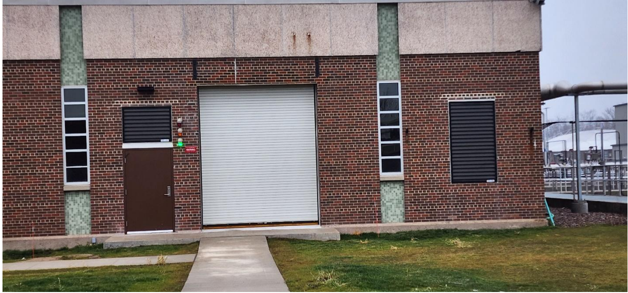
Louvre screens placed on south side of Structure 400 (Activated Sludge Building).
