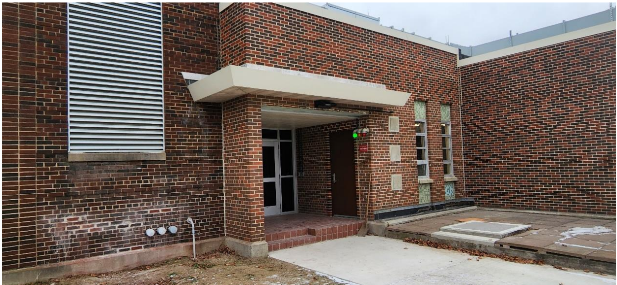
Structure 100 (Main Building) entryway front roof overhang completed.
