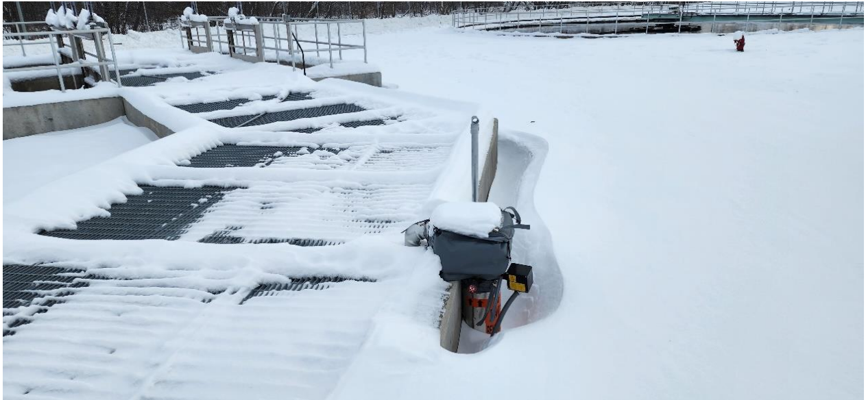
Phosphorus removal chemical (PRC) line insulation complete.
