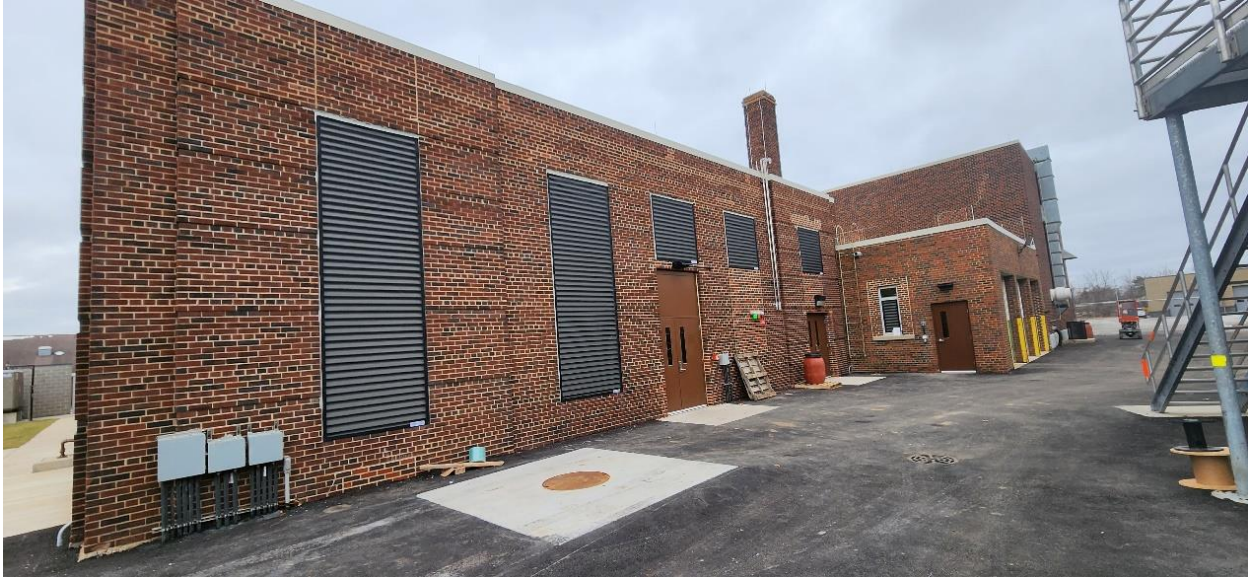
More louvre screens installed along east side of Structure 100 (Main Building).
