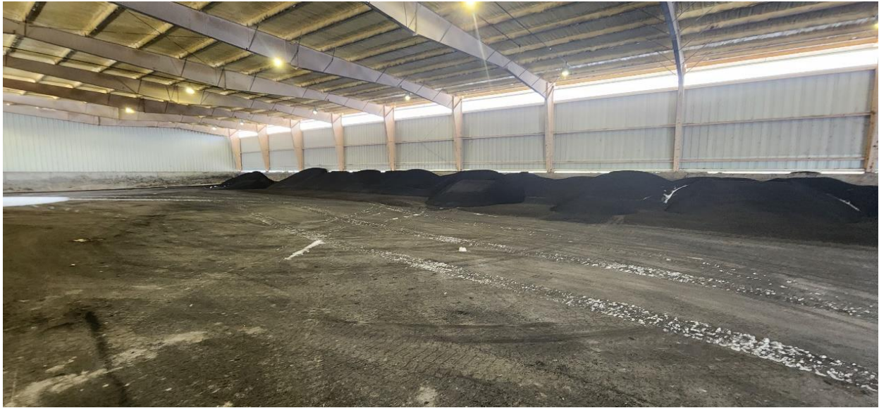
Biosolids Storage Building (Structure 760) in use.
