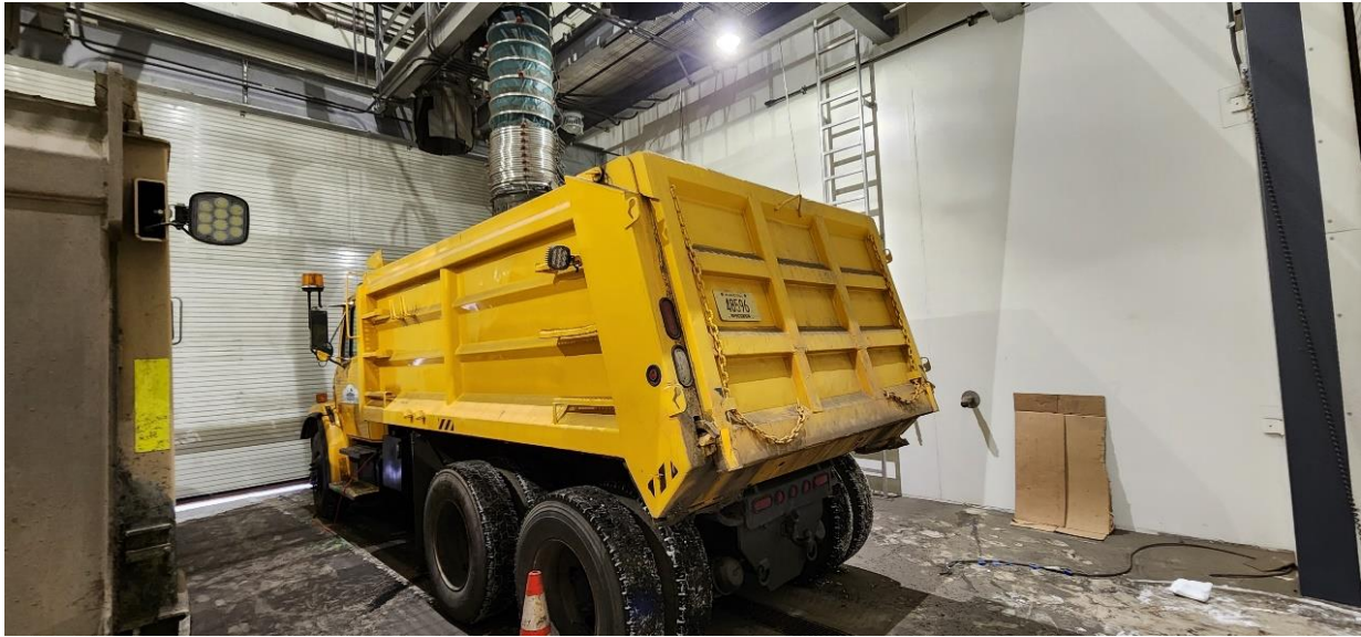
Biosolids chutes are fixed at Structure 770 (Solids Building).
