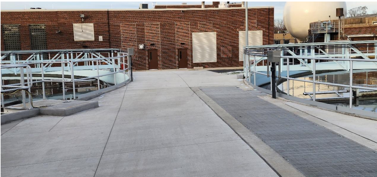
Kick plate on guard rails for Structures 310 and 320 (Primary Clarifiers 2 and 3).
