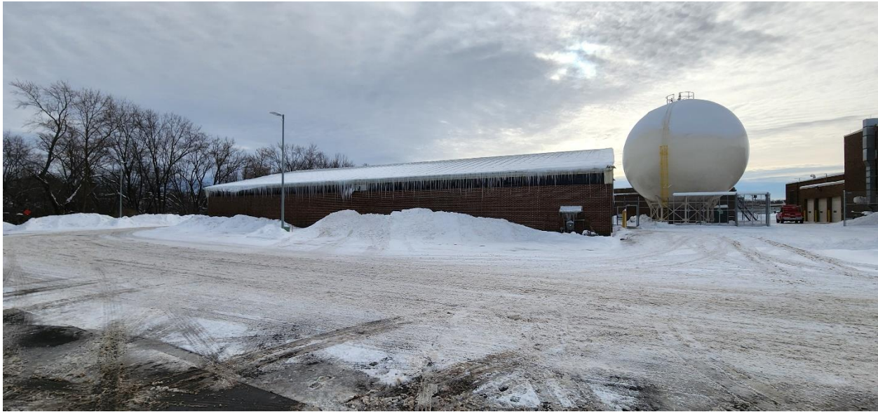
Parting Shots: Project is close to completion and no job trailers remain on a quiet winter day.
