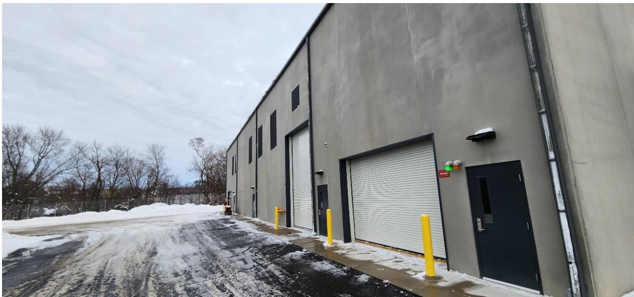
Louvre screens installed on north side of Structure 770 (Solids Building).
