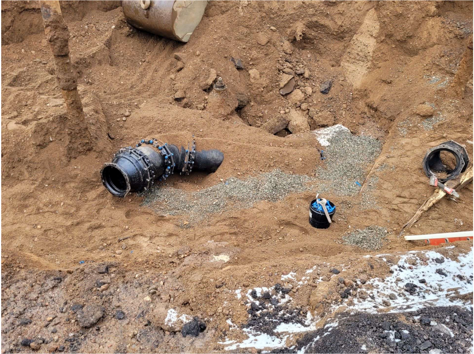
Final Connection of Well Piping to Bring Well 7 to New Facility
