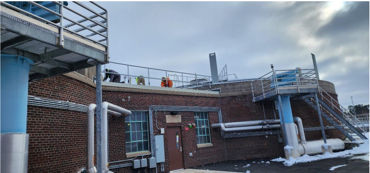
West hand/guard rail installed to proper height and membrane roof finished around railing at Structure 700 (Digester Building).
