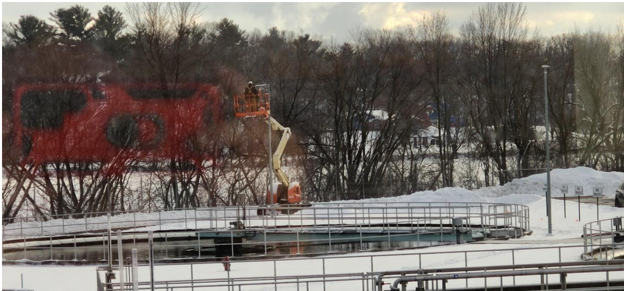
Working on finalizing yard lighting operation settings.
