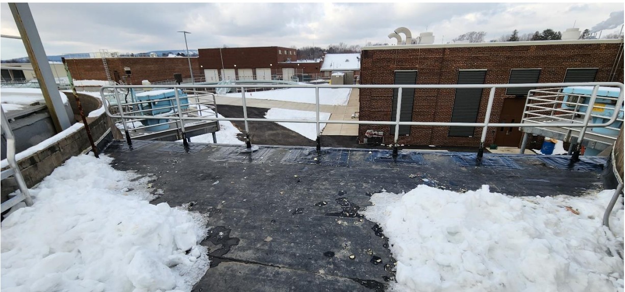
Membrane roof finished around railing at Structure 700 (Digester Building).
