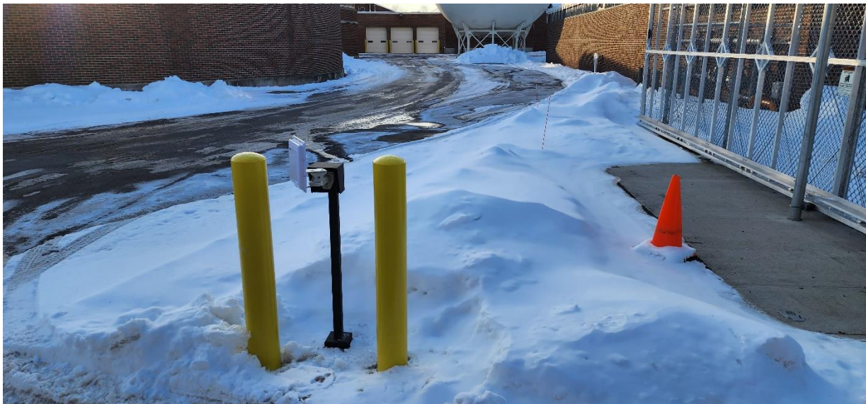
East gate card readers and electrical are installed.
