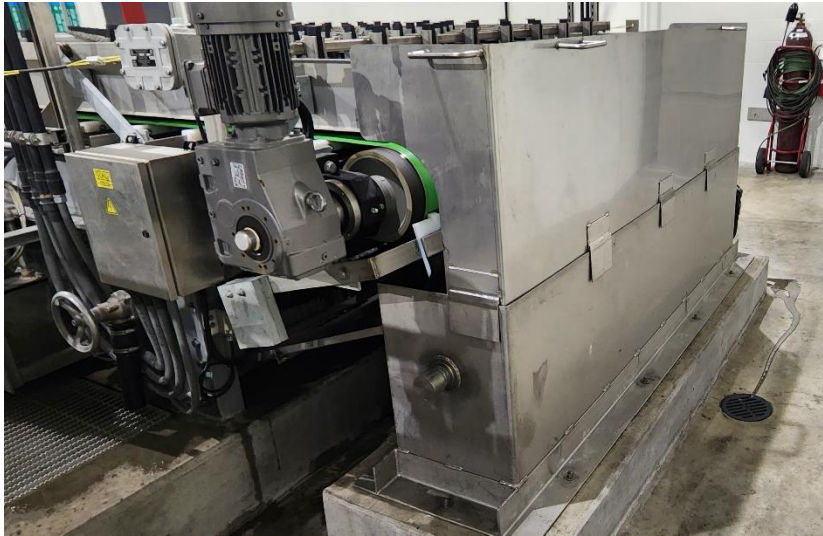
Left: Gravity belt thickener hopper extensions installed at Structure 770 (Solids Building).
