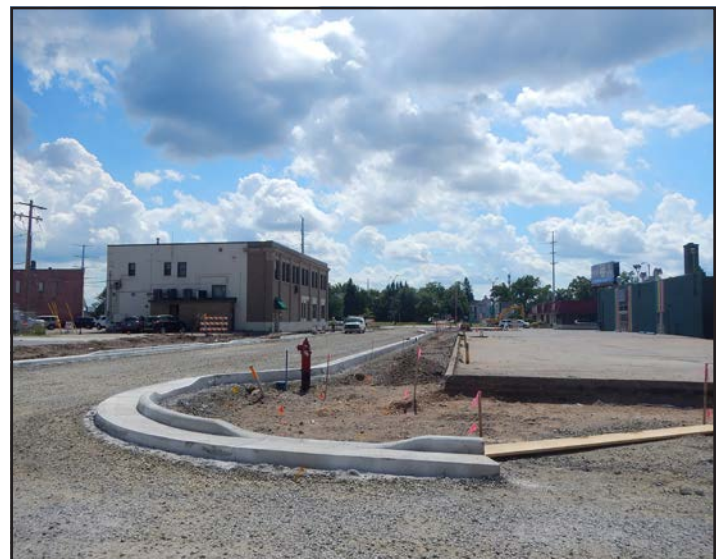
Reconstruction of 2nd Ave.
