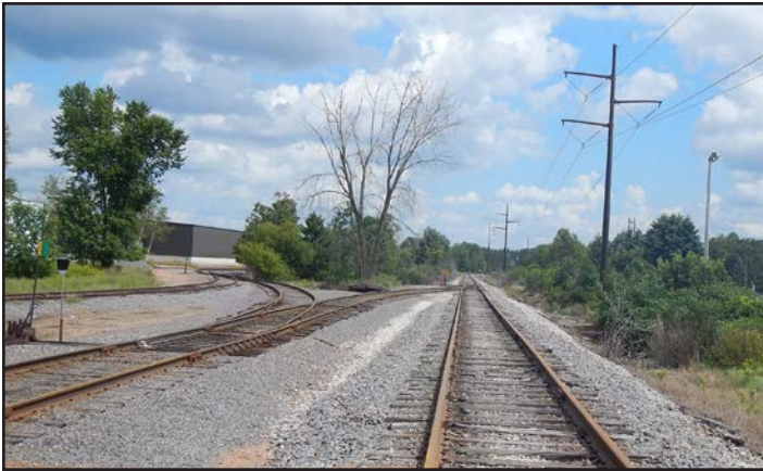
Rail lines in the Industrial Park.
