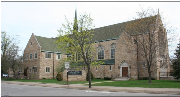
Zion Lutheran Church (1953), 709 N. 6 th Street.
