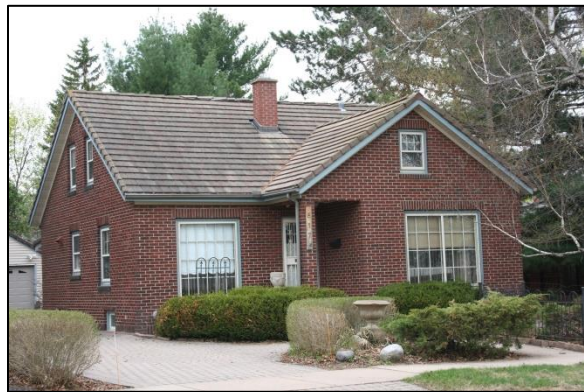
A circa 1947, Minimal Traditional house located at 817 Le Messurier Street.
