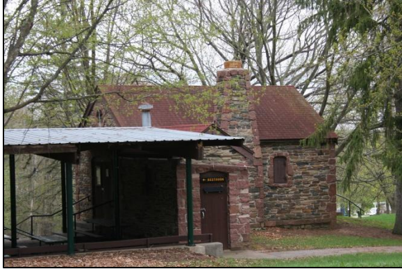
The shelter at Pleasant View Park (1940) is among a number of Rustic Style buildings in Wausau's parks.
