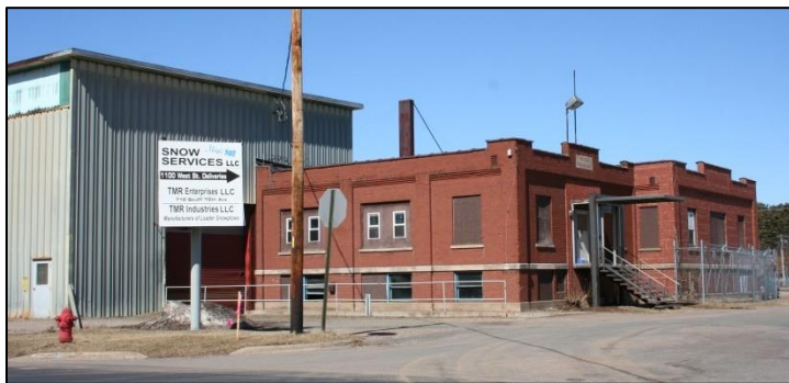
Wausau Iron Works (1910+), 738 S. 10 th Avenue.
