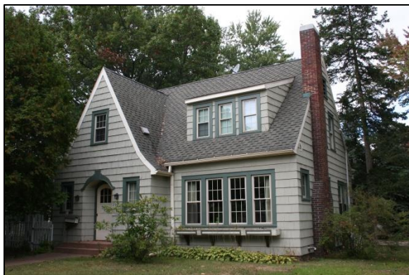
This Tudor Revival-style house at 202 Weston Avenue closely reflects the exterior appearance of ‘The Lynnhaven,’ a Sears, Roebuck & Company plan.
