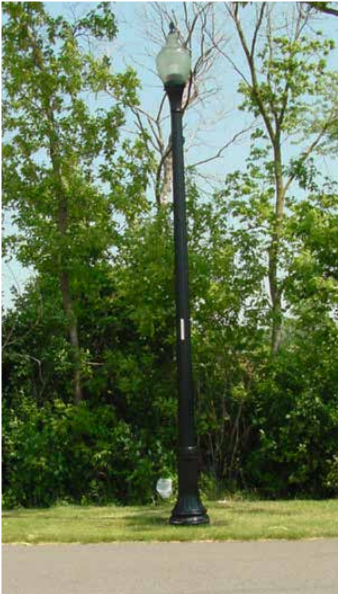
River Edge Parkway existing lighting
