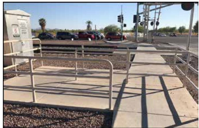
▲ Typical pedestrian maze barrier for public at-grade crossings and an example image of a maze crossing Image source: U.S. Department of Transportation, Federal Railroad Administration
