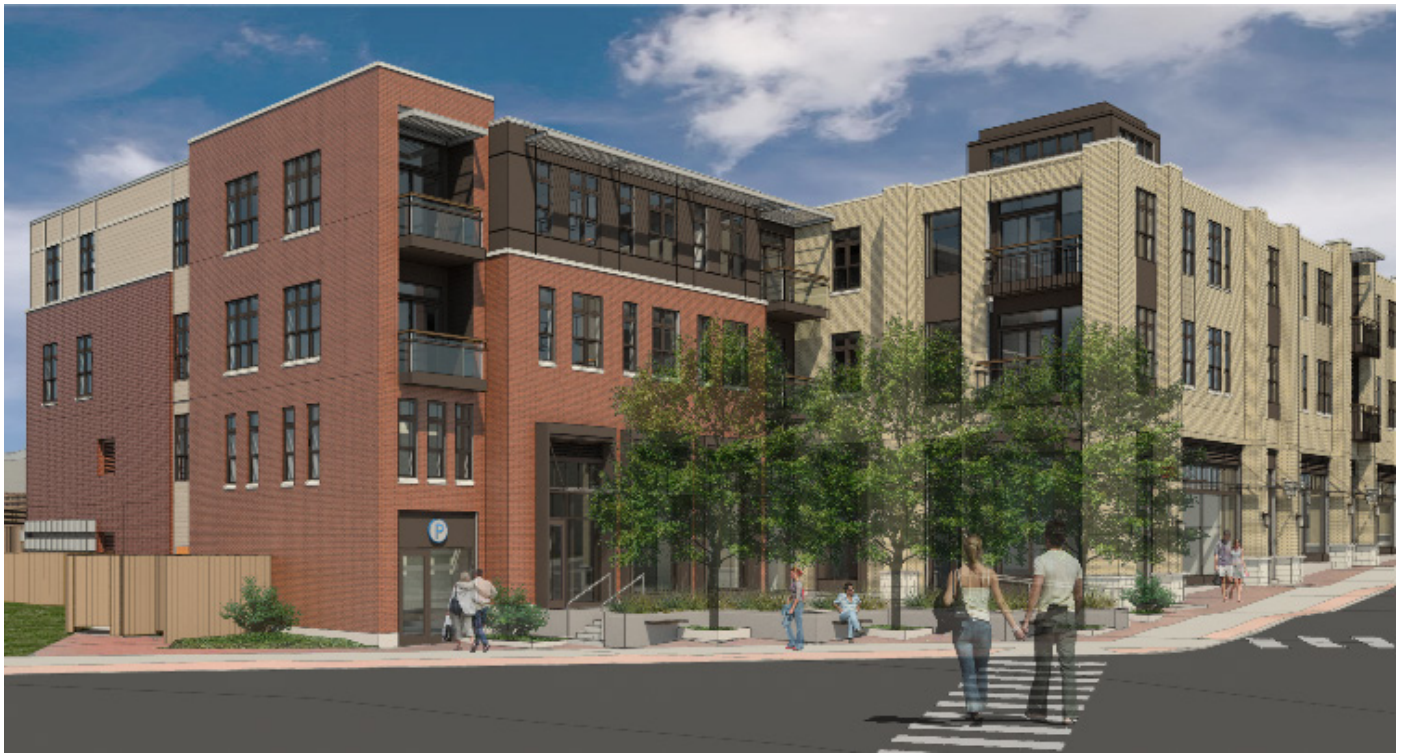
ABOVE: Harmonee Square, located in the village of Wauwatosa, is a three-story mixed use development that includes 30 apartments and 7,500 square feet of first-floor commercial space.
