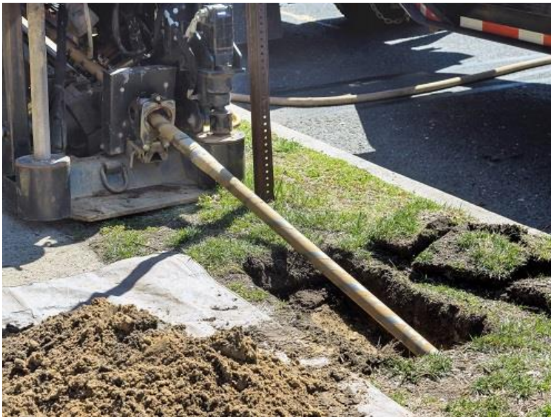
Figure 7-5: Surface Launched HDD Set-Up
