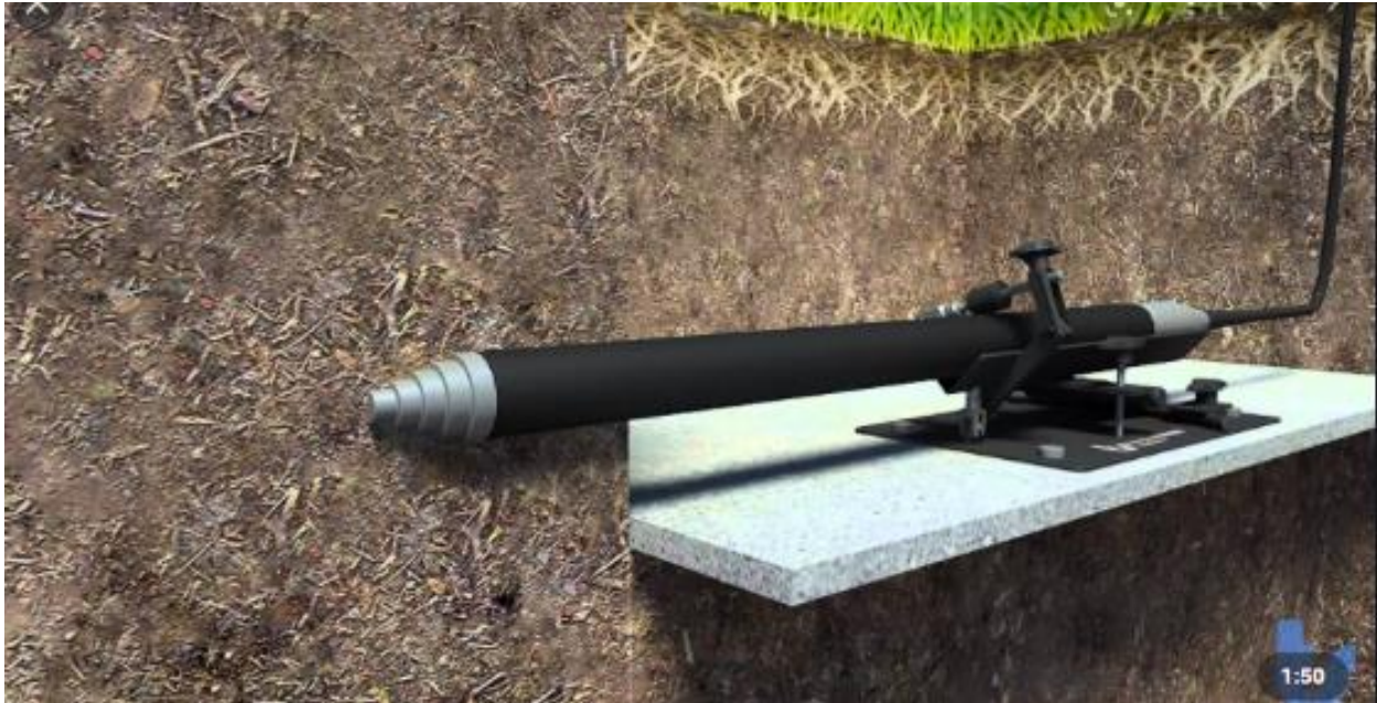
Figure 7-3: Example of a Horizontal Boring Tool Photo Courtesy of Trenchless Group
