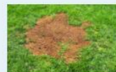
Temporary backfilled holes in your yard are filled with soil and left to settle.
