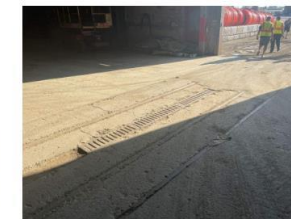
B. PREVIOUSLY REMOVED RAILROAD TRACKS THROUGH SITE
