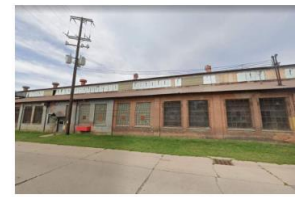
A. MAIN UTILITY LINE ENTRY TO SITE
