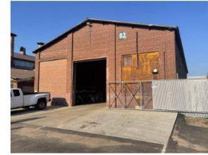
5. SHOP BUILDING 6,000 SF
